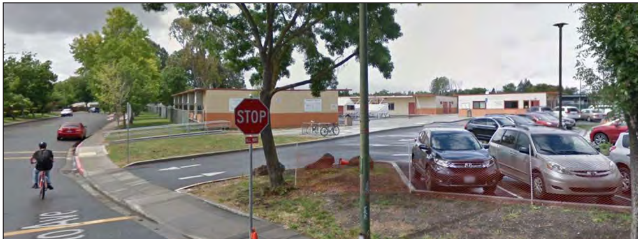
Montecito Preschool Site Frontage at Montecito Avenue
