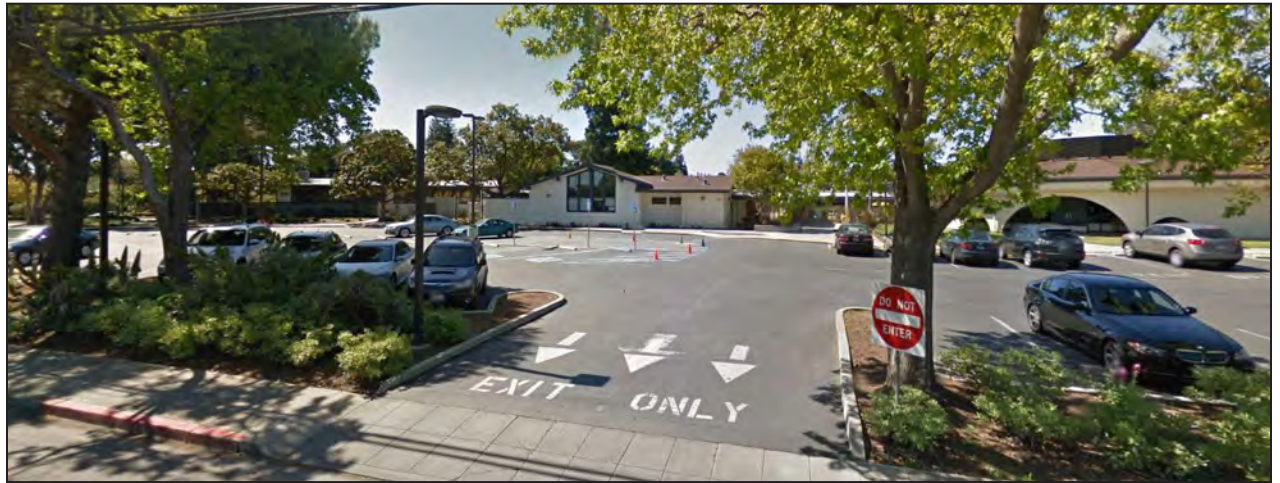
Slater (Google) School Frontage at Gladys Avenue
